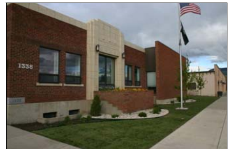
Completed service project
